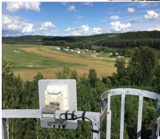
The Altai A8 Ein Super Wifi base station can deliver Wifi connectivity over distances of up to a Mile
