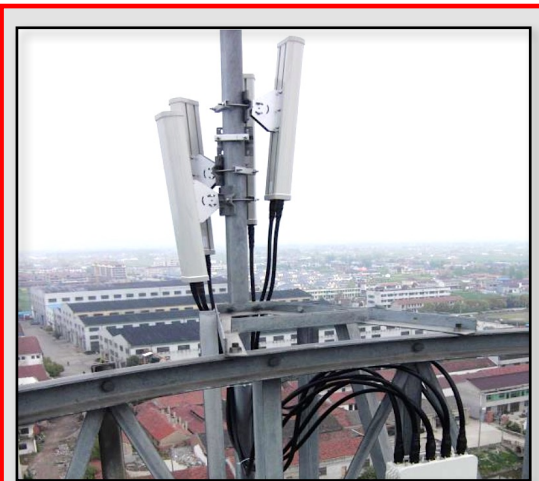
The Altai Technologies A8n Super wifi macro base station is a dual band radio supporting 2.4 and 5ghz bands delivering bi-directional connectivity to any standard wifi-enabled device over distances of up to 3/4 mile while supporting 255 concurrent data sessions and 1000+ associated connections.
